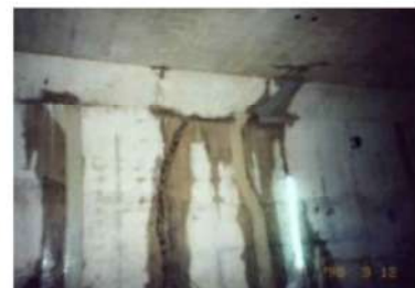
Impact from groundwater level recovery to the subway (Groundwater leakage)
