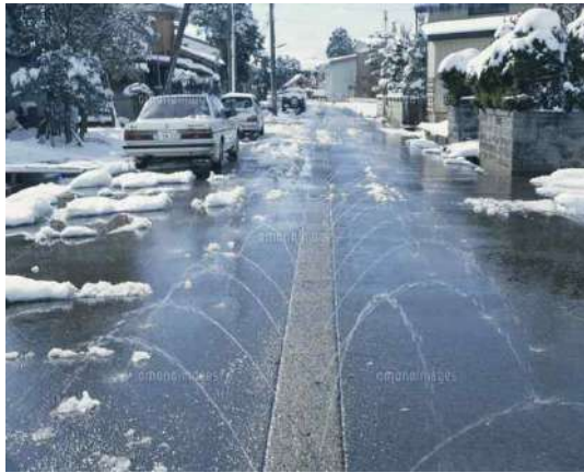
Photo 1 Snow melting system using groundwater
