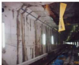
Impact from groundwater level recovery to the subway (Groundwater leakage)
